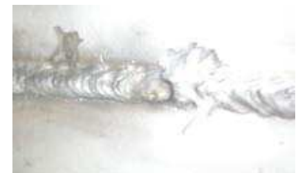
a) a pinhole on liner weld, the result of an arc impact after the electrode was removed
