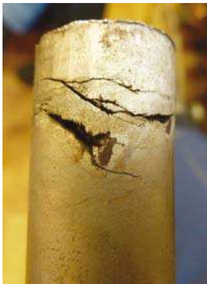
e) cracks in a tube from the tube sheet area
